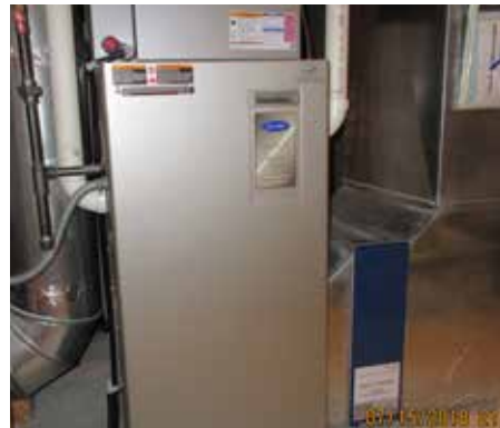
Figure 2: 90% Condensing Gas Furnace
