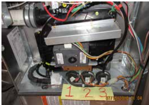
Figure 4: 96%, Three Stage Gas Furnace
