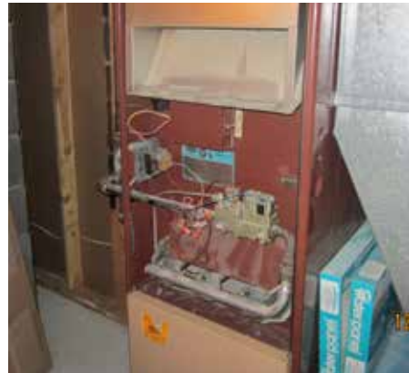
Figure 1: Naturally Drafted 60% Gas Furnace
