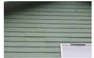
Figure 6: Loose Siding
