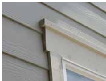
Figure 9: Trim installed over siding
