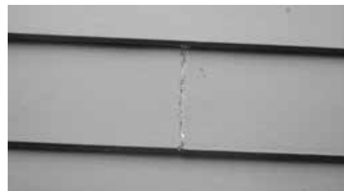
Figure 1: Caulked Butt Joint
