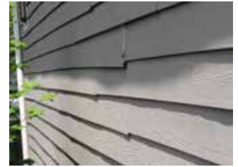
Figure 5: Loose Siding
