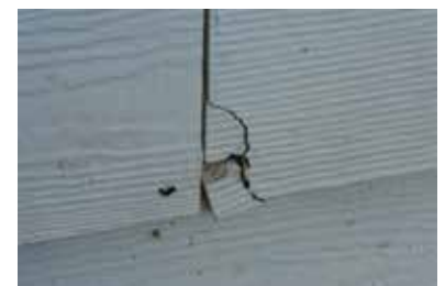
Figure 12: Cracking Corners
